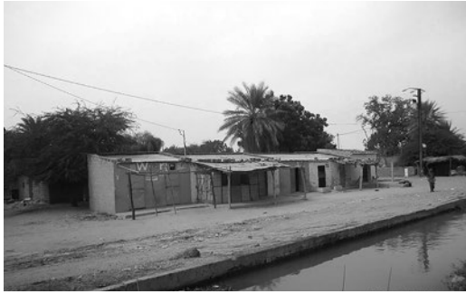
Guédé Chantier and the central canal that enables farmers to irrigate their rice fields.
