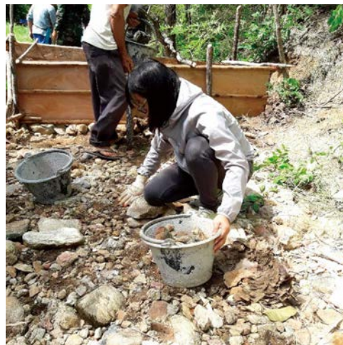
The volunteers were divided into many groups. Some helped collect rocks from the ground, while others helped pass the rocks into the check dam.
